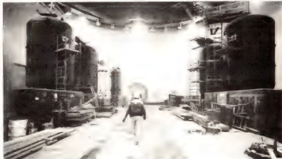
Steam generators at the abandoned Marble Hill power plant near Madison, Ind.
